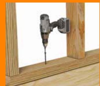
BOTTOM PLATE TO FLOOR JOIST
