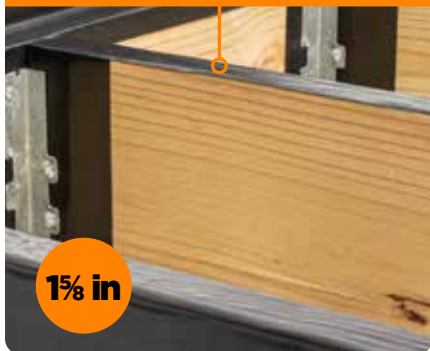
TOP OF JOISTS
