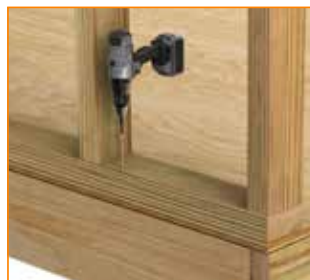
BOTTOM PLATE TO RIM BOARD
