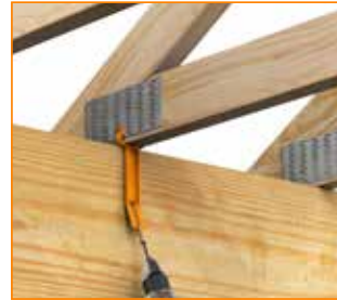
BEAM TO TRUSS
