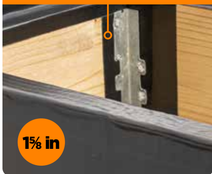
BETWEEN JOIST HANGERS AND LEDGER BOARD
