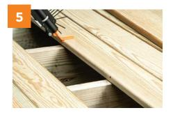
**FASTEN EVERY JOIST** Install a screw at every joist on the outer edge of the board.
