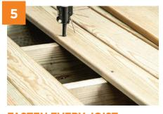
**FASTEN EVERY JOIST** Install two screws at every joist until the entire board is installed.
