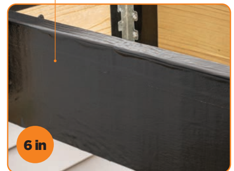
F BETWEEN RIM JOISTS AND FASCIA
