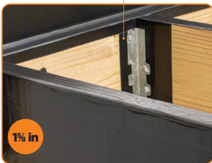
A BETWEEN JOIST HANGERS AND LEDGER BOARD
