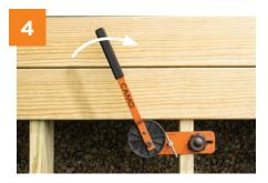
**CLOSE THE GAP** Keep turning until the board is in desired fastening position.
