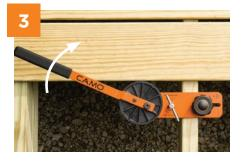
**BEGIN BENDING** Apply pressure by moving the handle towards the deck board.
