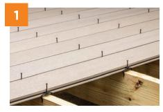
PREPARE BOARDS Lay down multiple rows of boards and CAMO Universal Deck Clips.
