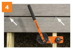
**FASTEN** Leave LEVER in place until all clips are fastened.
