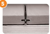
Slide the clips (screws and gussets) down the groove, positioning one over each joist on both sides of the board.
