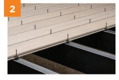
**REPEAT ALONG THE BOARD** Place a clip at every joist along the length of the board.
