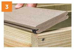
PLACE BOARD Tilt board up slightly to set it in the clips.
