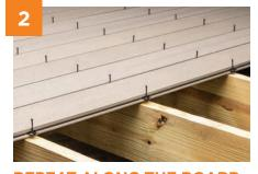
**REPEAT ALONG THE BOARD** Place a clip at every joist along the length
